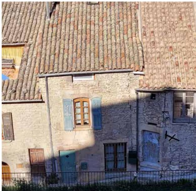
MAÇONNERIE DE MOELLONS CALCAIRE CLAIR
