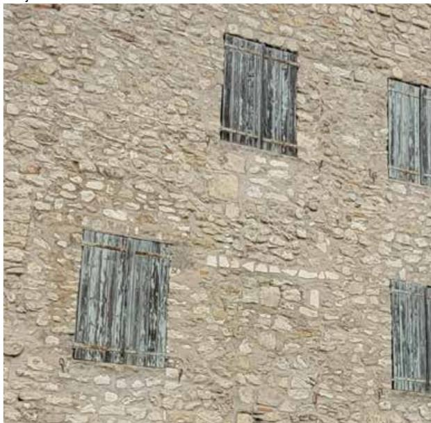
MAÇONNERIE DE MOELLONS CALCAIRE DORE
